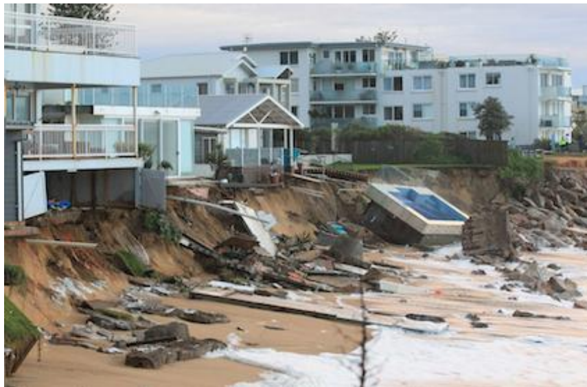
Figure 1 This figure shows severe coastal erosion at Collaroy-Narrabeen Beach (June 2016).
