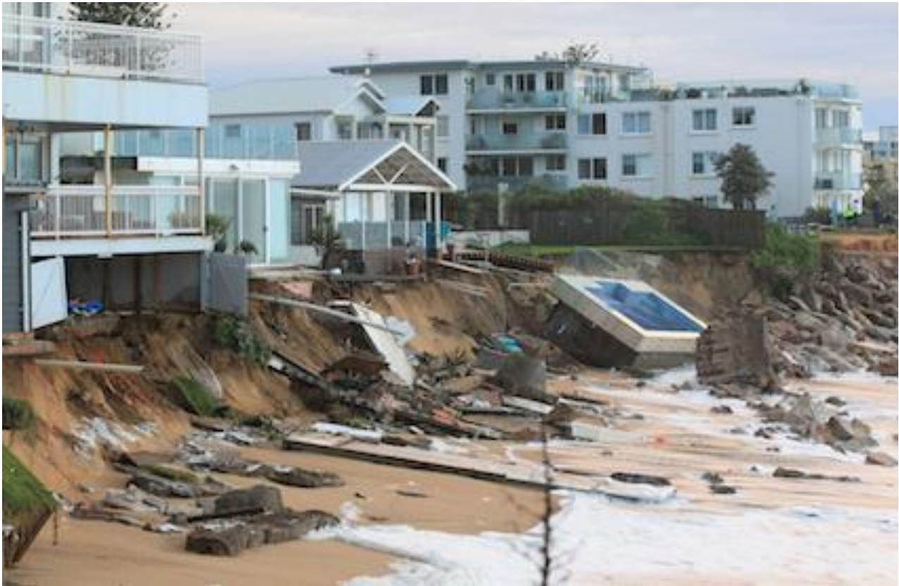
Figure 3 This figure shows severe coastal erosion at Collaroy-Narrabeen Beach (June 2016).
