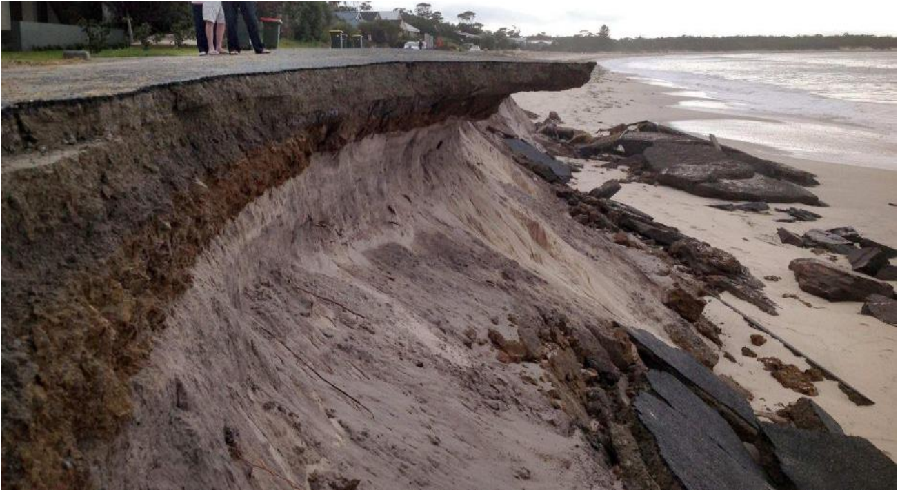
Erosion at Jimmy's Beach, NSW
