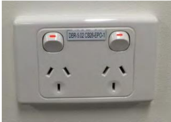
Figure 7 – General non-essential 10A outlets (non-generator back-up)
