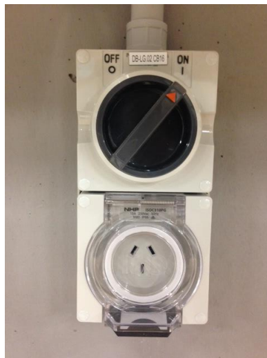
Figure 6 – Weatherproof plug sockets
